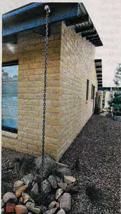
Violet Town in bloom Vasili visits the market (top) and sees chainwire replacing conventional downpipes (above).
